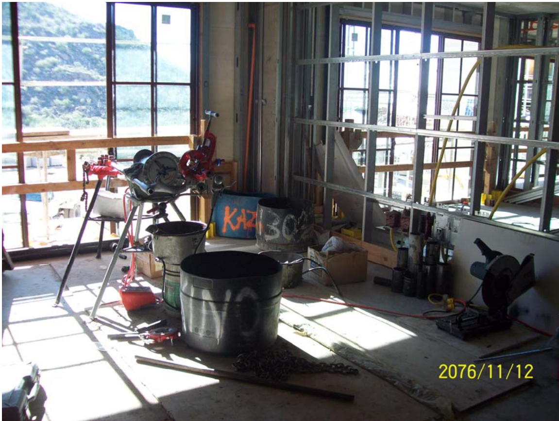
Housekeeping on the jobsite is very important
